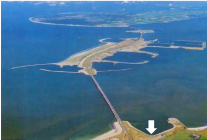
Figure 11.10.2. Intake location at arrow, Oosterschelde storm surge barrier (structure in center) Photo: Pinterest.
