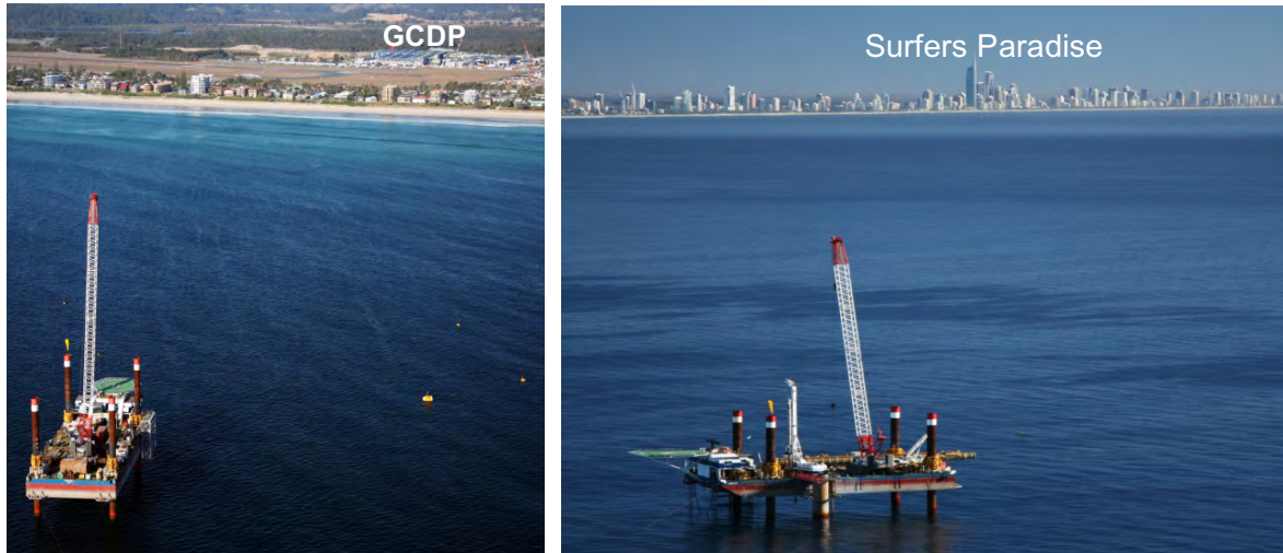
Figure 11.12.2. Self-elevating platform over intake during construction with the GCDP in the background (left) and Surfers Paradise (right).
