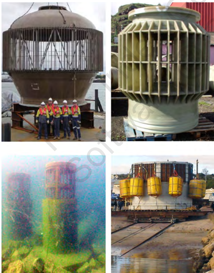
Figure 6.9. Various offshore intake heads. From top left, clockwise to bottom left, courtesy of WaterSecure, Increa, Water Corporation, and Abengoa.
