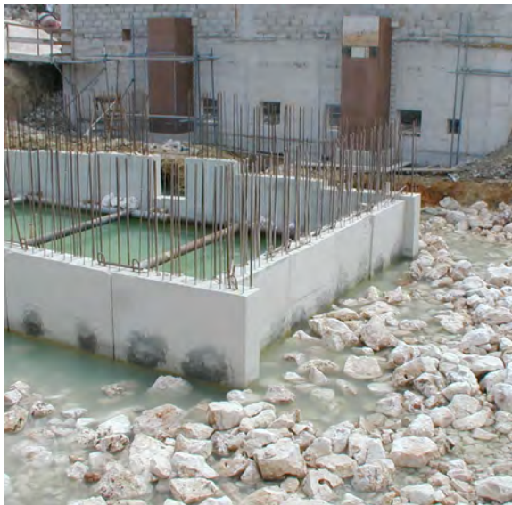
Figure 6.27. Karst pit intake system. Photo: T. Pankratz.
