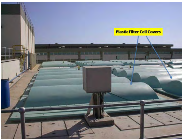
Figure 9.20. Gravity filters protected with plastic covers for control of algal growth showing covers of gravity filters in Ashkelon, Israel.
