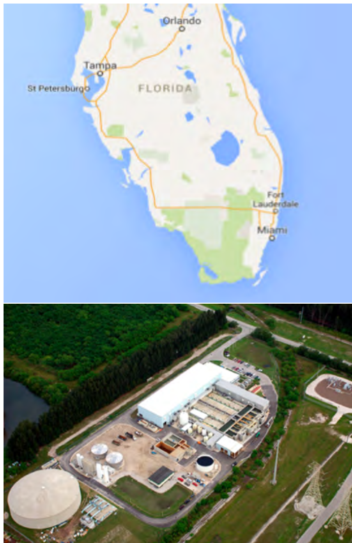
Figure 11.9.1. Location of the Tampa Bay Seawater Desalination Plant (top) and aerial view (bottom; Accessed on 11 Nov. 2016 http://www.accionia.us/projects/water/desalination-plants/tampa-bay-desalination-plant/ ).
