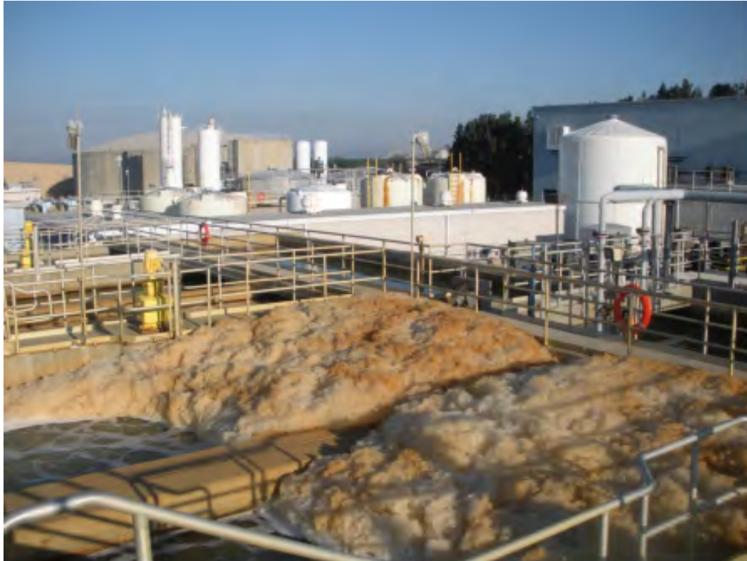
Figure 11.9.4. Foaming observed in the rapid mix basins during pretreatment at TBSDP. Source: Voutchkov (2009).
