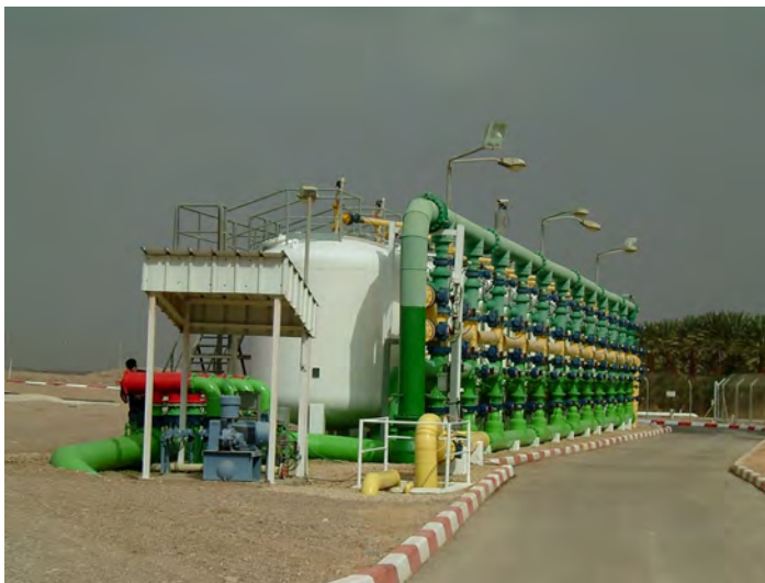
Figure 9.22. Vertical pressure pretreatment filters capacity. Photo: Voutchkov 2013.
